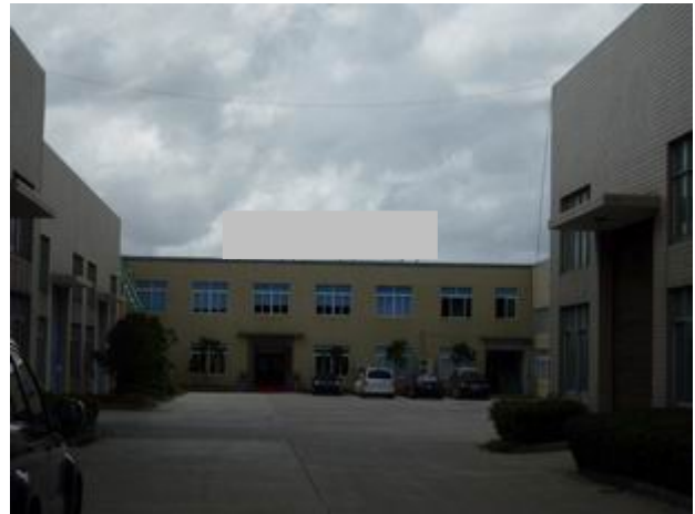
Factory exterior view
