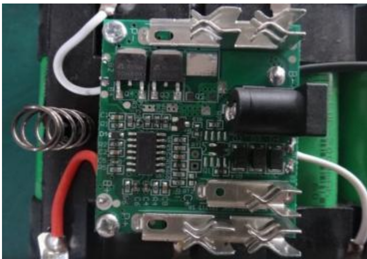
Internal workmanship and critical component check
